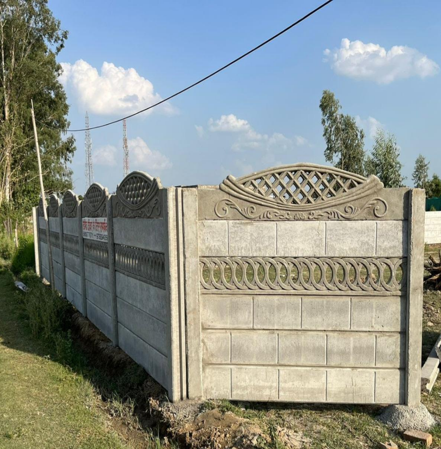
HANDMAD PRICAST COMPOUND WALL
